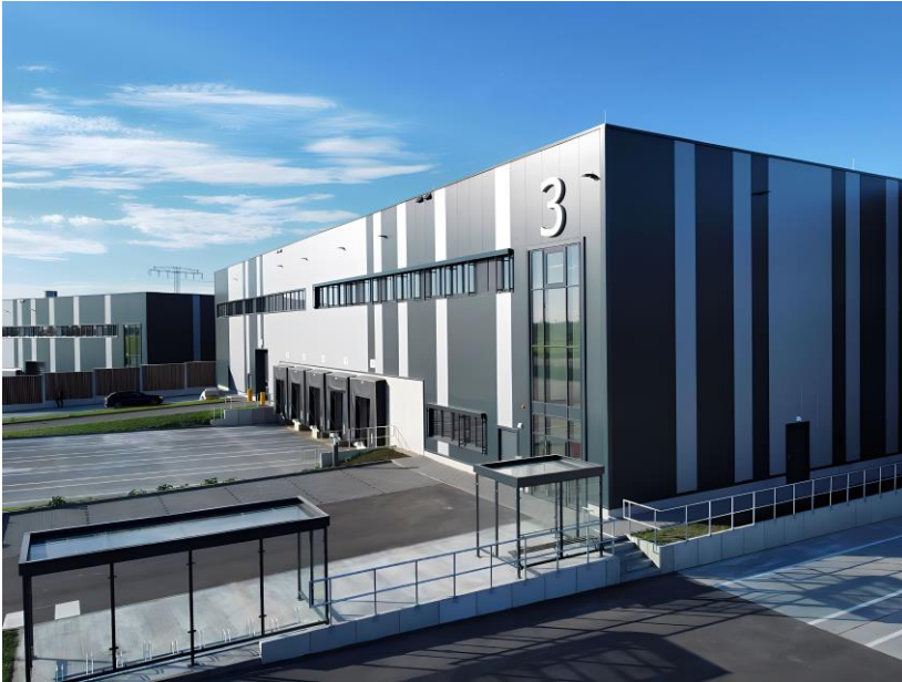
New logistics building in Leipzig
